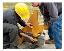
Note: On smaller rail it may be necessary to lift up the front end of the stop an inch or two in order to get the bolt clamps into position.
